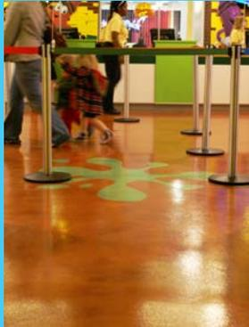
Following the repair of the substrate, a white primer was applied to provide a uniform under coat for the Key Luster Metallic base. Once cured, the fun began as the creative installers with **Durex** were allowed to make their colorful magic. The KEY LUSTER METALLIC was spread by trowel and then backrolled in an artistic figure eight pattern over the wet resin. This technique provided a cloud like appearance in the metallic bronze colored basecoat.
