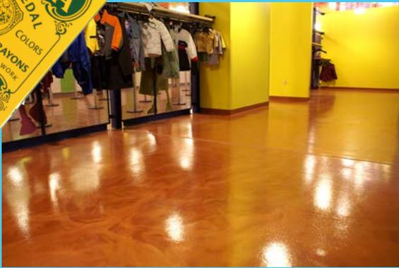
The *Crayola Experience* lobby renovation started with the removal and relocation of walls. Following this, **Durex Coverings** began the flooring installation by removing an existing resinous floor down to bare concrete. Significant patching was required to level and smooth the substrate where wall and posts once existed.
